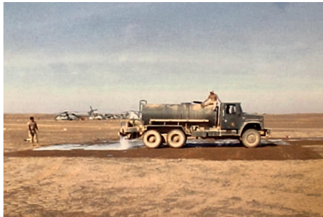
Rhino Airfield: "Rhino Snot" used for Helo Pad Dust Suppressant. Photo taken by IT3 Martin Reiger.
